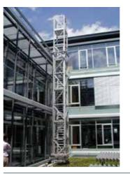
With box ladders it is possible to safely climb inside the ladder. The box ladder can traverse easily with an electrical motor or manually along the tracks mounted on the building.
