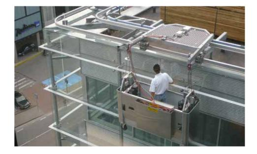
A light roof trolley is an extremely flat machine traversing on two parallel tracks. The roof trolley consists of one or two suspension jibs. The suspension jibs can be either foldable (with fixed outreach from the facade) or telescopic (adjustable outreach). With both suspension alternatives, the jibs are moved out of sight when the roof trolley The Roca roof trolley is the is not in use.
